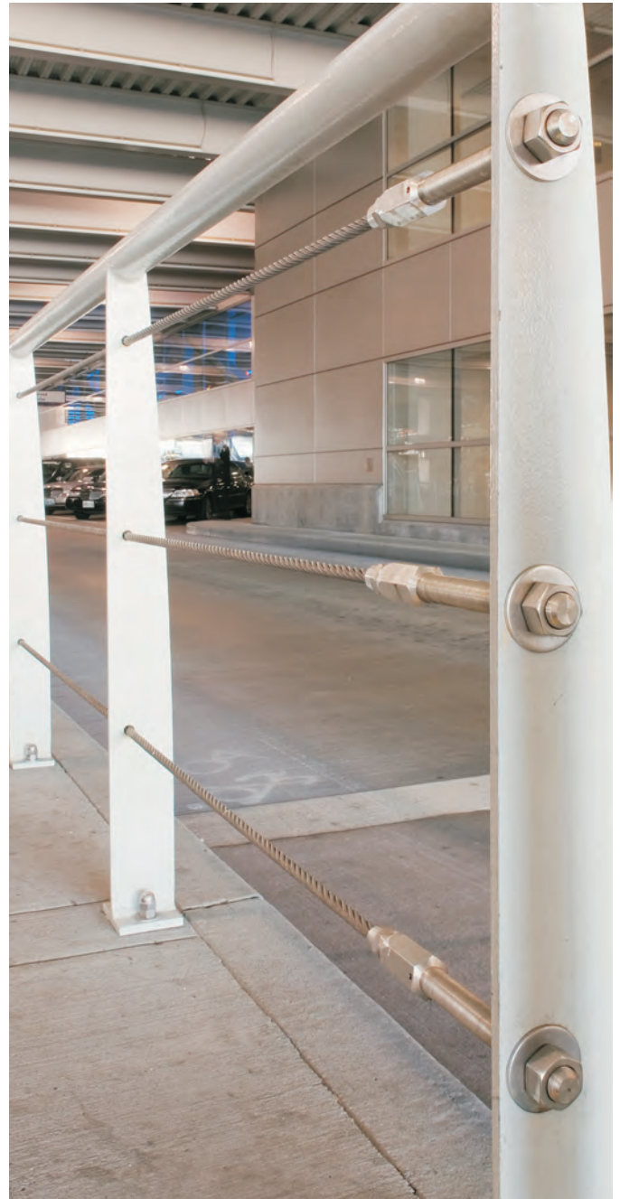
Stud Fitting - Pedestrian Walkway - Portland International Airport
